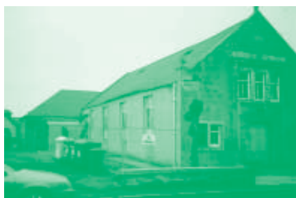
Memorial Hall prior to demolition.
